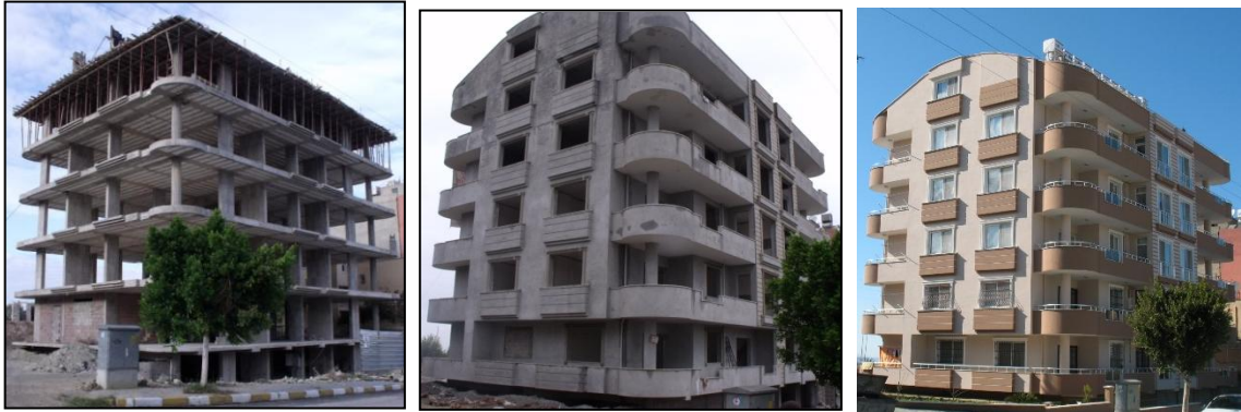
Fig. 1. without infill walls Fig. 2. with infill walls Fig. 3. under usage
